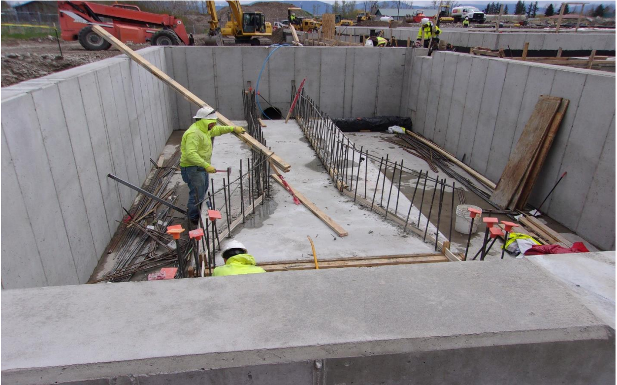
Inside the formwork for the headworks splitter structure - intricate and complex.
