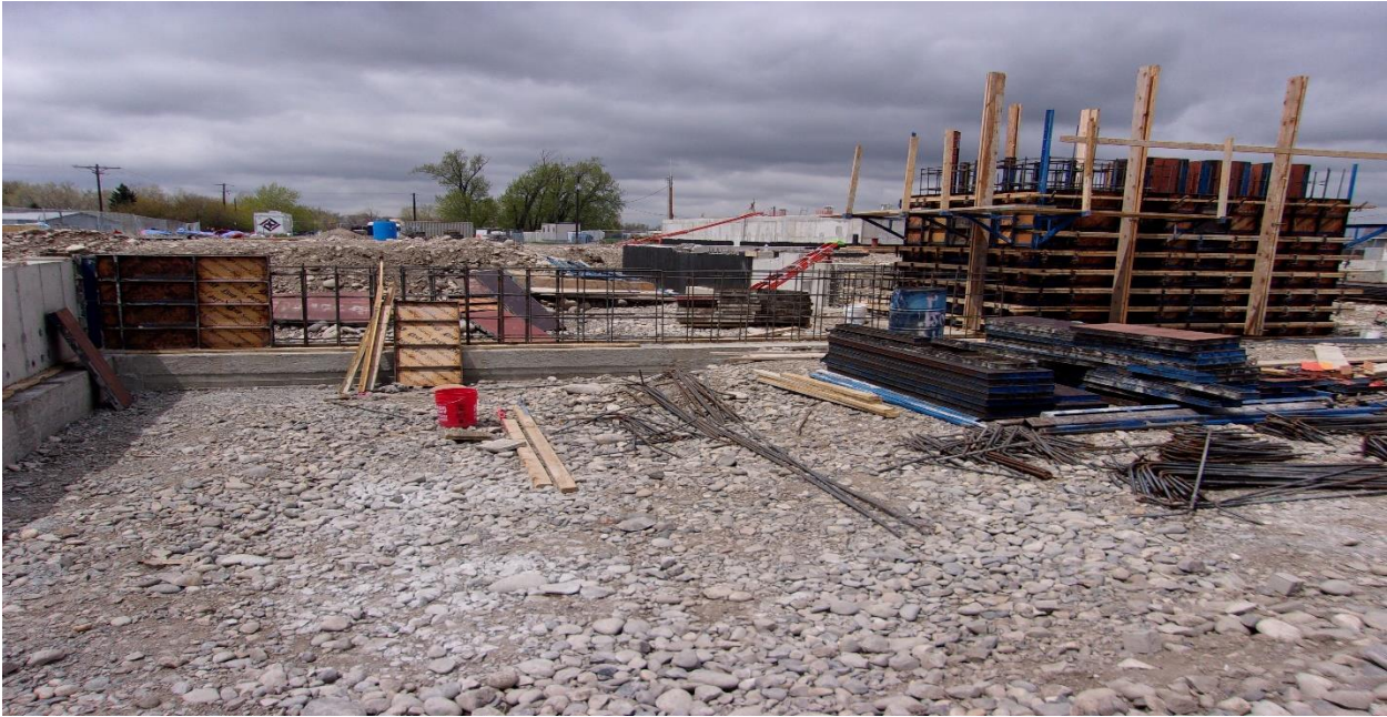
Splitter Structure form work.
