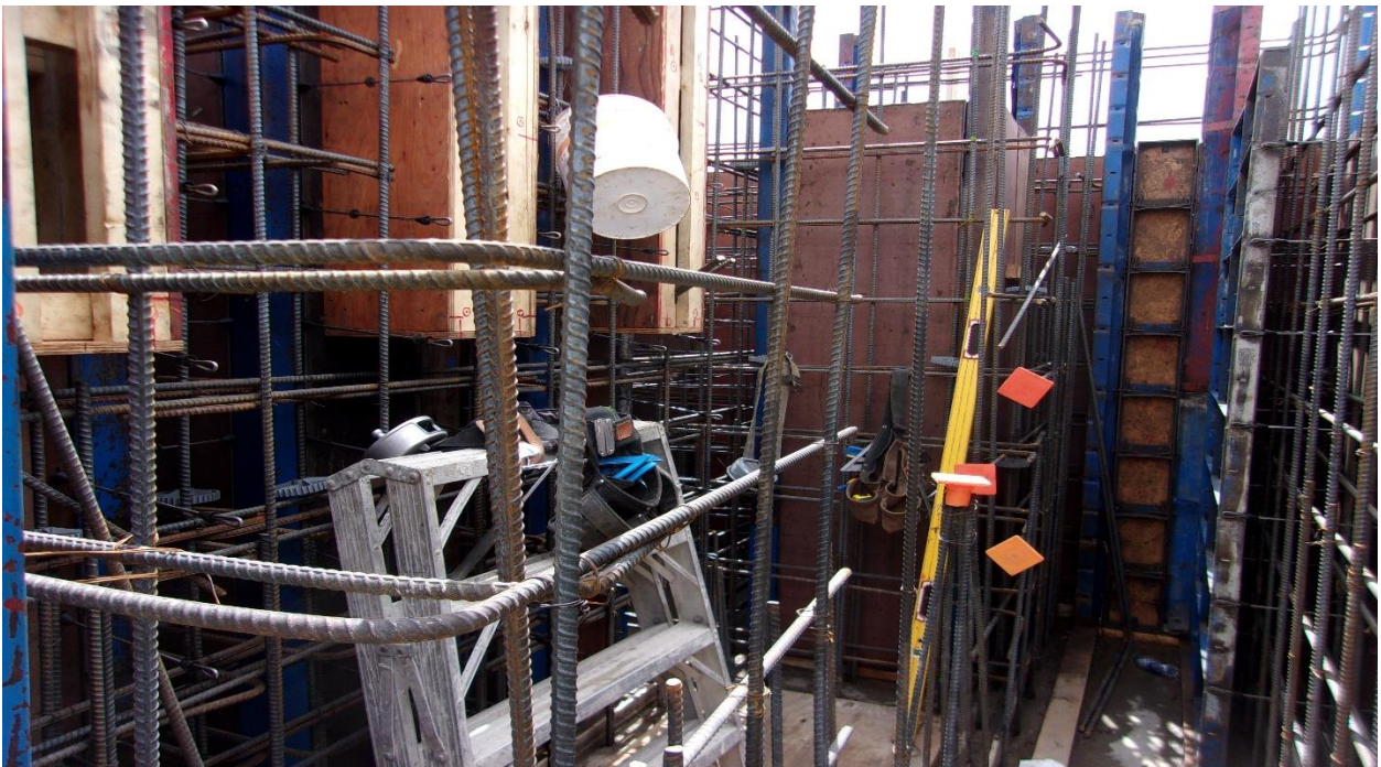
Inside the formwork for the headworks splitter structure - intricate and complex.
