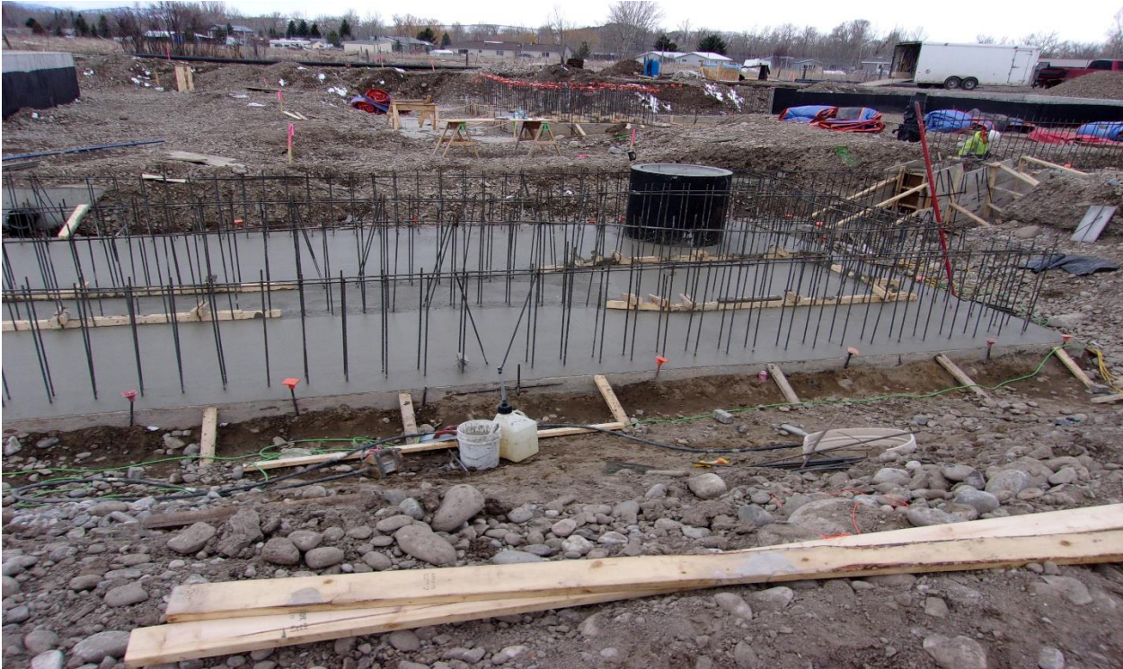
UV Raceway First concrete placement.
