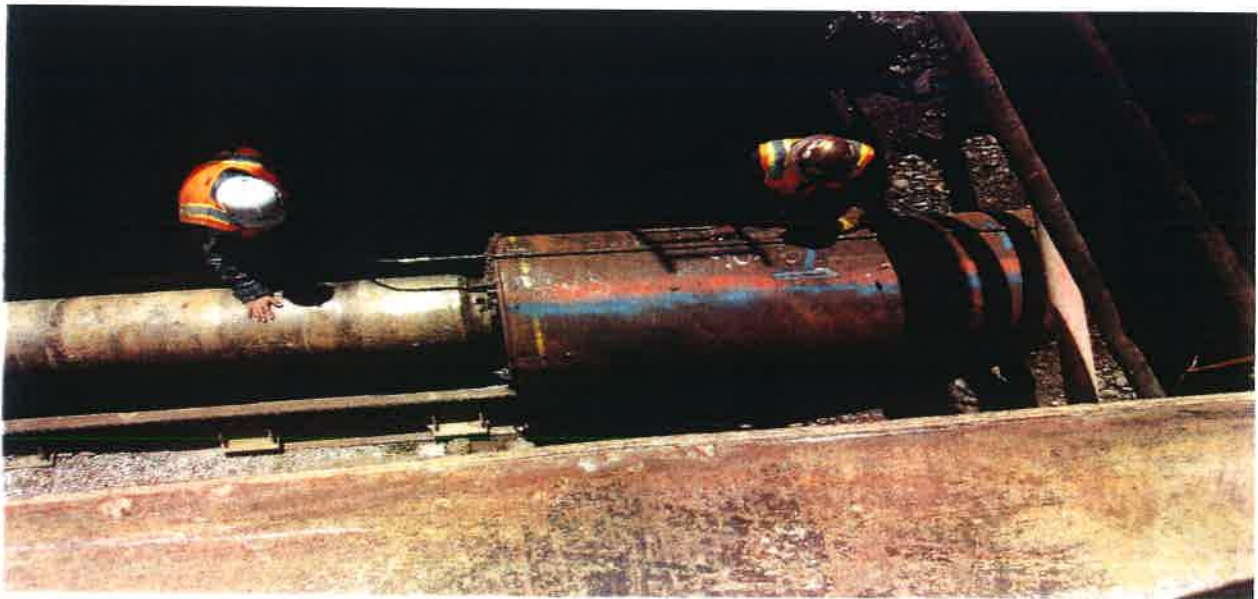
Air Hammer Driving 42" casing
