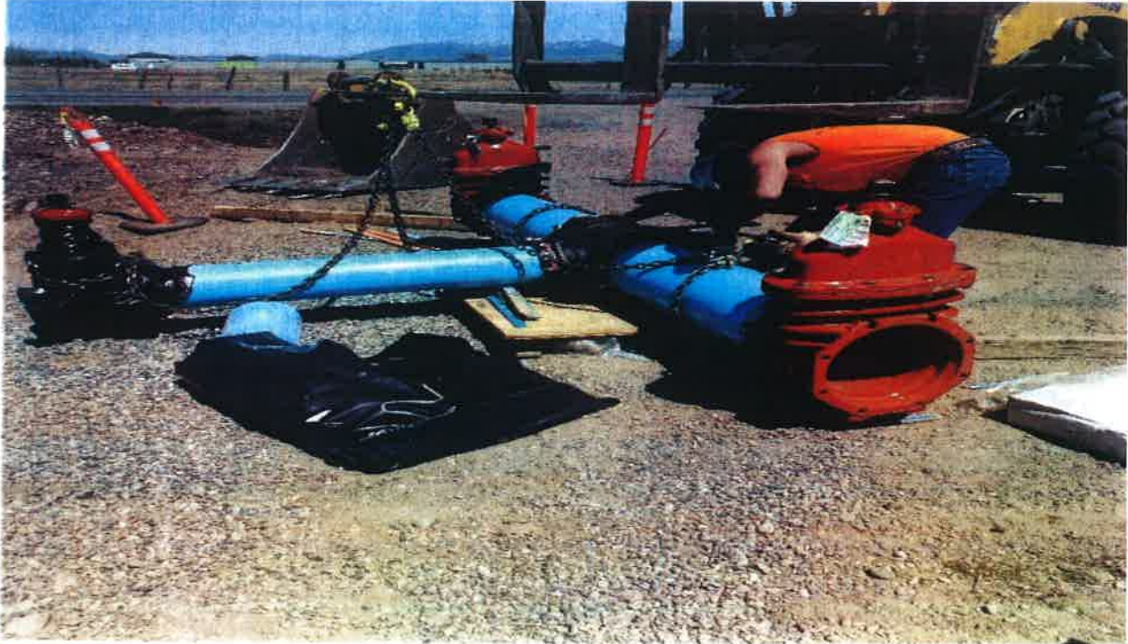
Assembling Water line fittings for installation
