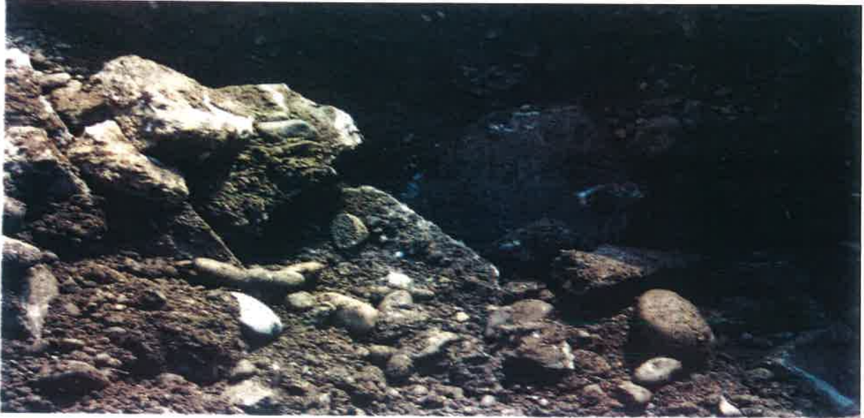
Concrete in excavation
